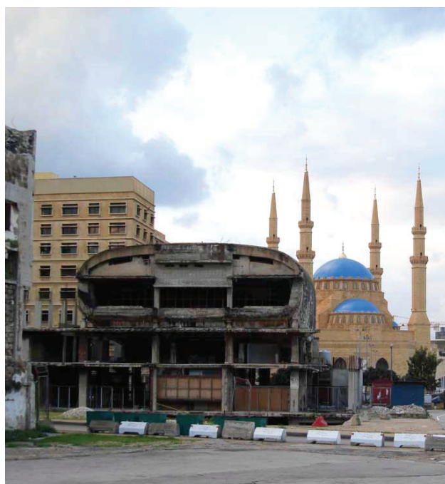
The Mohammad Al-Amin Mosque establishing a new scale in Beirut's city centre and on the edge of the still unbuilt Martyrs' Square.
